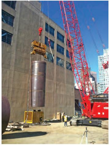
4100 Crane with 200-6 vibratory hammer holding 120" diameter x 30'0" long casing to be installed in Bent 5.
