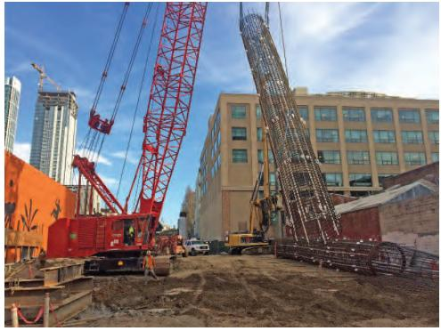
Rebar cages being hoisted into the air with limited clearance from nearby properties.
