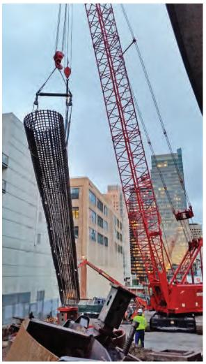
Rebar cages being hoisted into the air within only a few feet clearance from neighboring properties.
